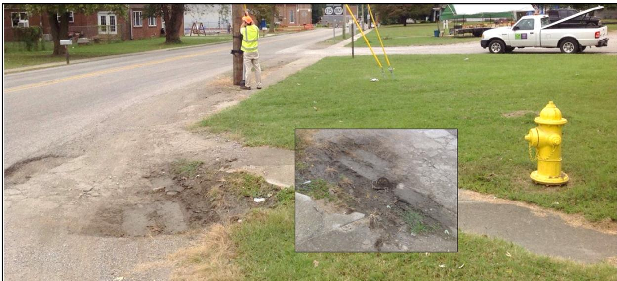
Figure 21: US 41/KY 115 Intersection Sidewalk and Close-up of Damaged Water Main Cover
